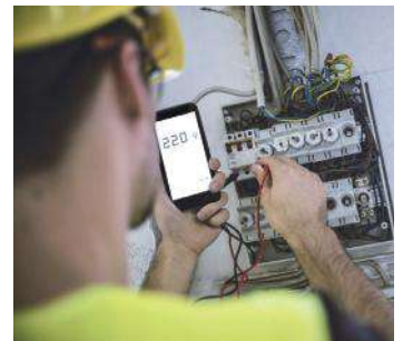
Electric Power Inspection
